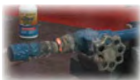
Cool Gel protects surfaces when welding
